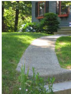
A pervious asphalt walkway is an attractive addition to home landscaping.
